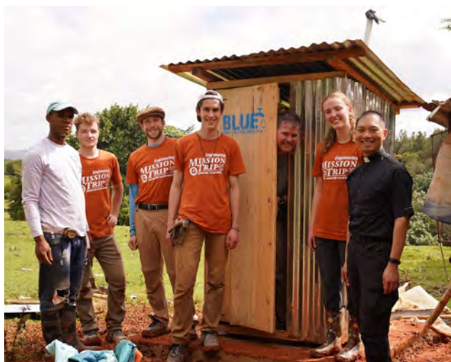
Engineers Building Latrines in Dominican Republic
